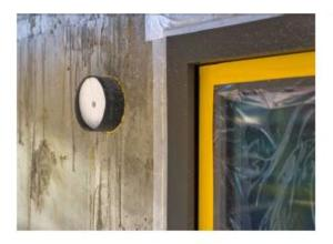
The facade elements of the LUNOtherm series are combined with the Silvento ec concealed clamp vents and the ALD external wall inserts.
